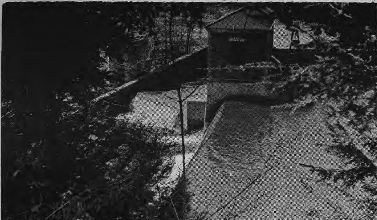
This dam at the southern end of Greenwood Lake controls the flow into Wanaque Reservoir.
