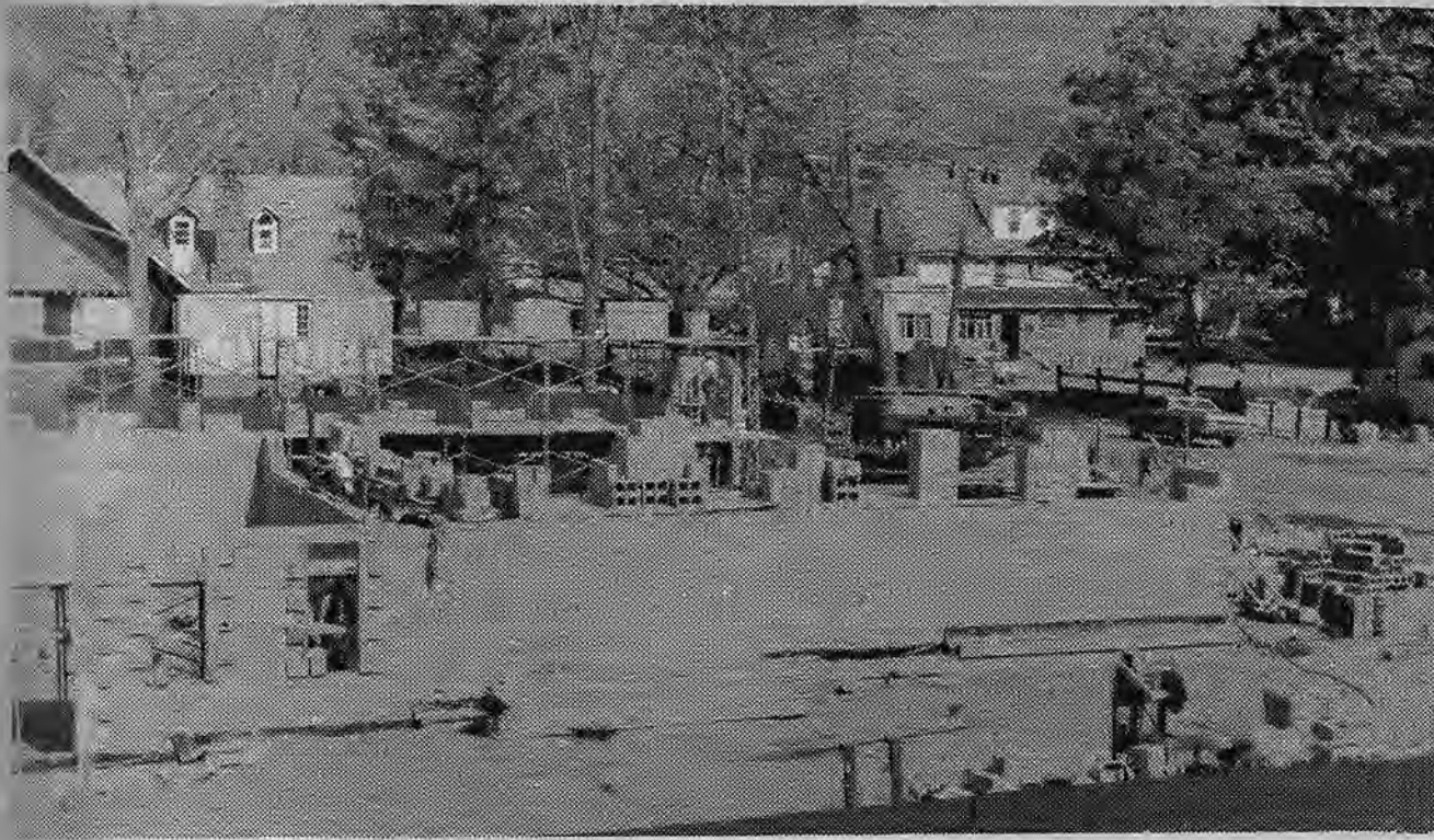
The new Firehouse and Village Offices under construction during the 1970s.
