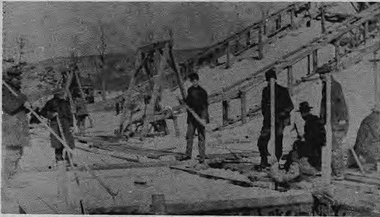
Cutting ice at Greenwood Lake, N.Y. The Mountain Ice Company had two commercial ice houses on the east shore which held 90,000 tons of ice. The wooden structures in this picture were "troughs". The ice was slid up these structures and into the ice house.
