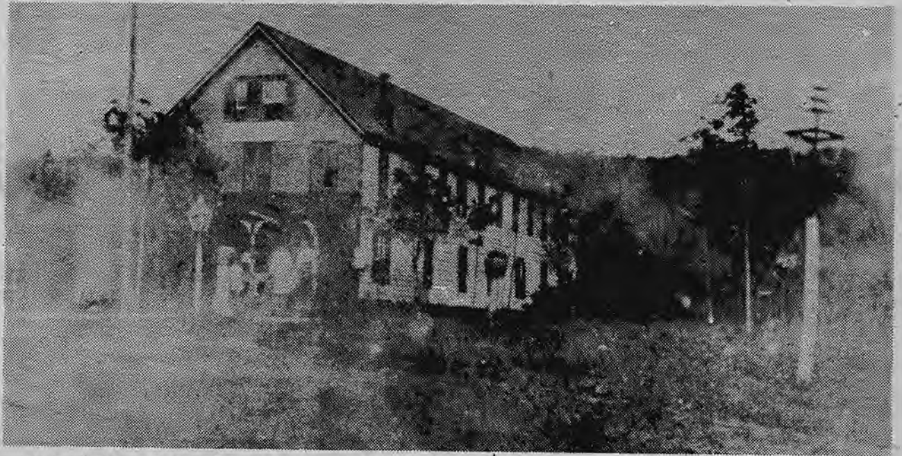
Marr and Hazen's Arcade on Oak Street and Windermere Avenue (Yellow Submarine). The sign over the door reads "Billiards - Bowling Alley." (The bowling alleys were upstairs!) The building was sometimes used as a village meeting hall.
