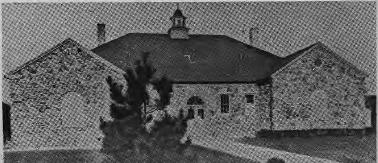
The stone school house was built in 1927. It was added to in 1950; five additional rooms, the auditorium and the cafeteria were built. Another addition was put on in 1961.
