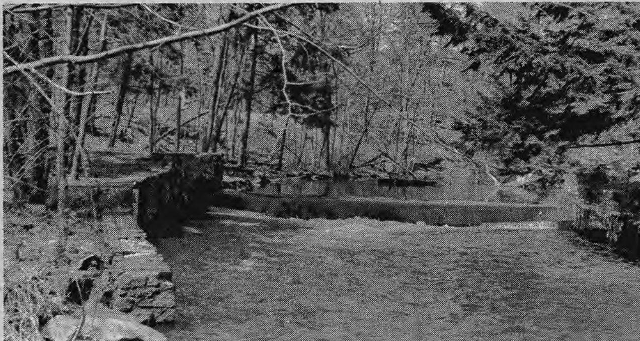
Evidence that Greenwood Lake's waters have been dammed more than one is supplied by this photo of a smaller dam just nearby the watershed dam.
